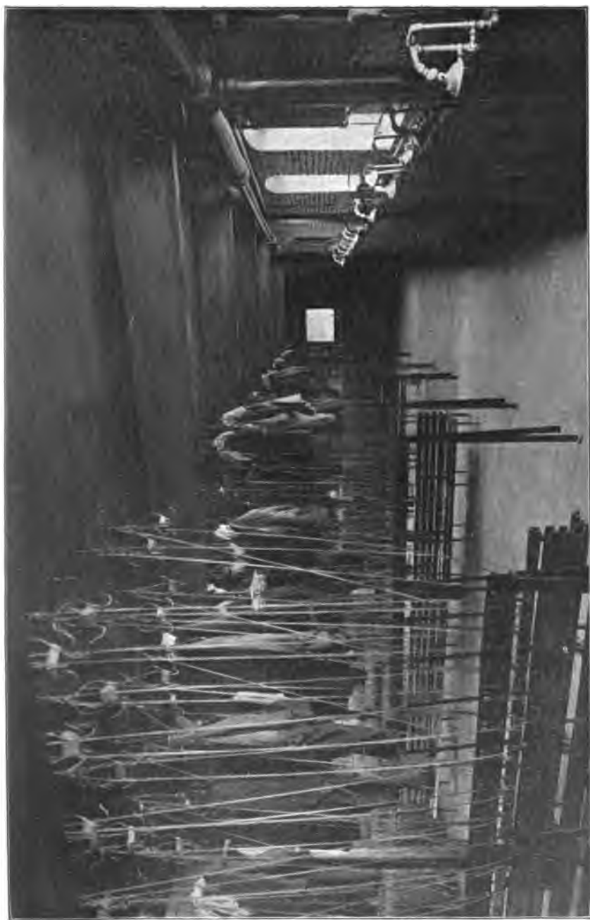
Fig. 2. Change House at the Marianna, Pa., Mine, of the Pittsburg-Buffalo Coal Co.
